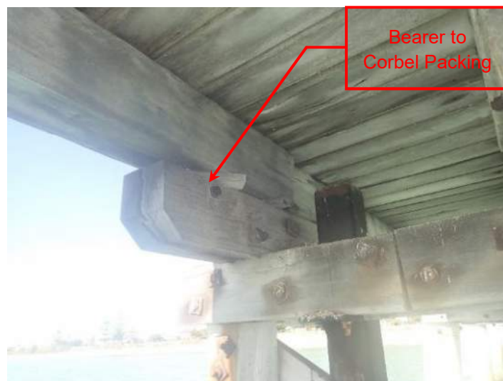
Figure 43 – Typical Bearer and Corbel Timber Packing
