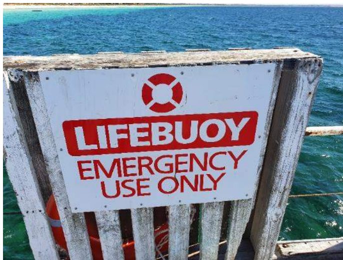
Figure 34 – Typical Condition 4 Sign (Defect: Weathering)
