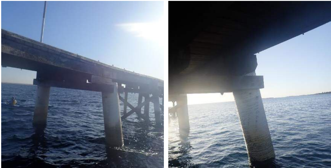
Figure 44 – Raking of Concrete Piles
