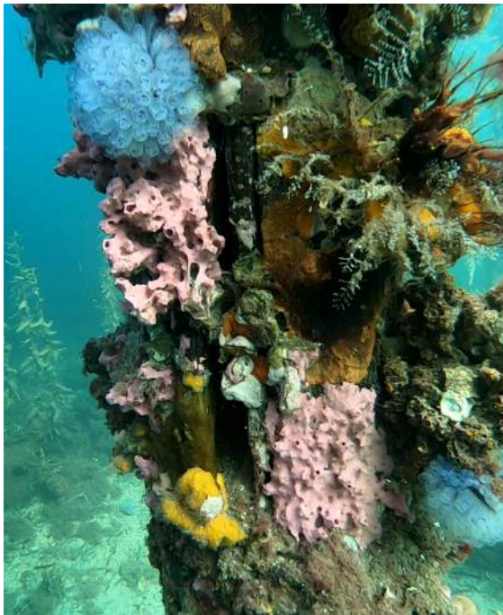
Figure 8 – Typical Condition 6 Timber Pile (Defect: Necking & Splitting)
