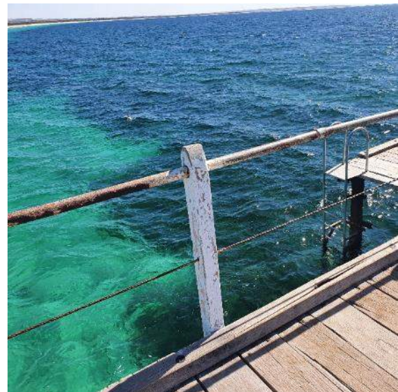
Figure 30 – Typical Condition 4 Handrailing (Defect: Surface Corrosion)
