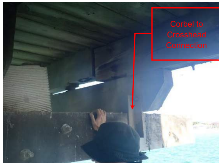
Figure 42 – Typical Bearer to Crosshead Connection
