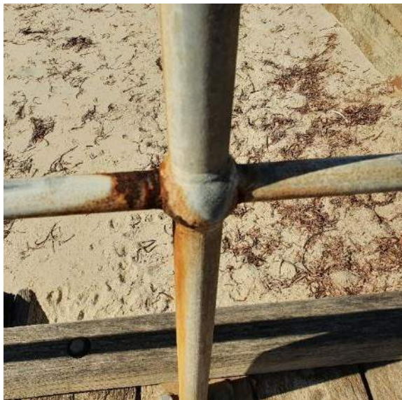
Figure 30 – Typical Condition 4 Handrailing (Defect: Surface Corrosion)
