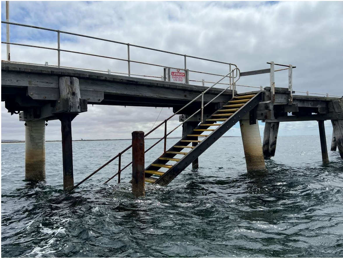
Figure 57: Jetty Ladder between bent 24 and 25
