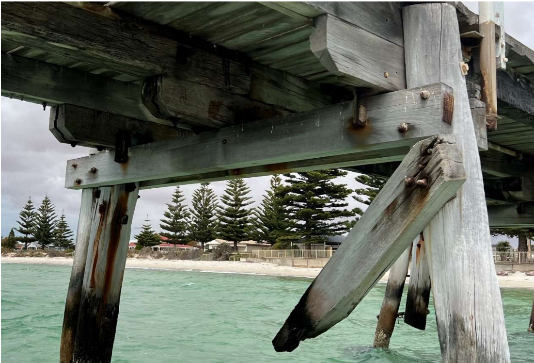
Figure 40 Typical condition '7' corbel
