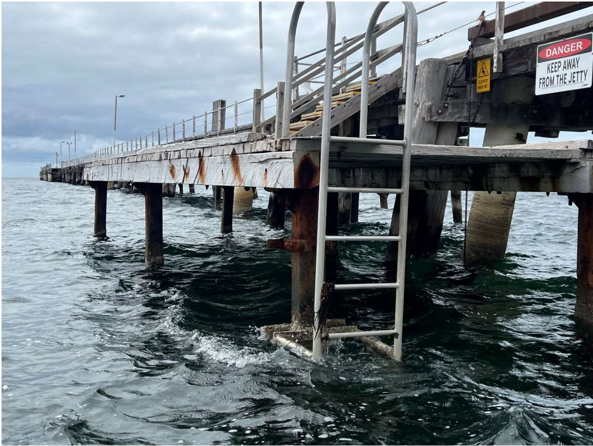
Figure 55: Lower Landing Dive Ladder
