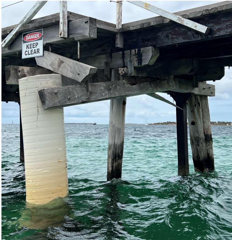
Figure 22 Typical Condition '7' Concrete encased timber pile
