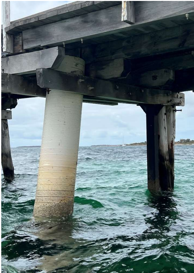
Figure 20 Typical Condition '4' Concrete Encased Pile
