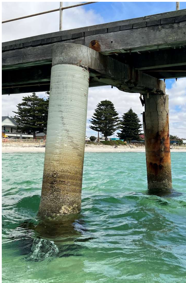
Figure 21 Typical Condition '5' Concrete Encased Timber Pile
